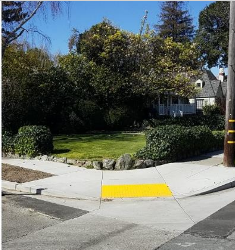
COMPLETED ACCESSIBLE CURB RAMP
