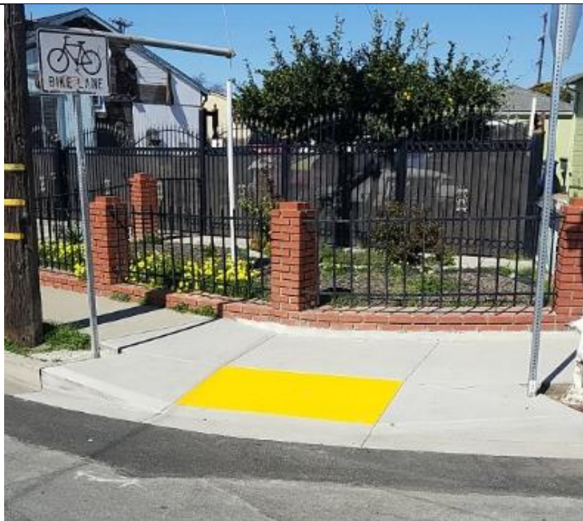
COMPLETED ACCESSIBLE CURB RAMP
